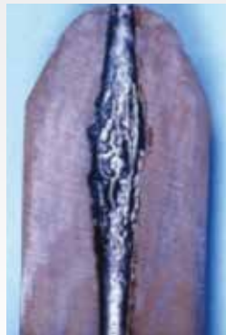
Erosion and corrosion
